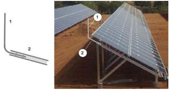
Fig. 2. Nonisolated L.P.S in PV applications. (1) Aluminum air termination rod. (2) Connection clamp.
